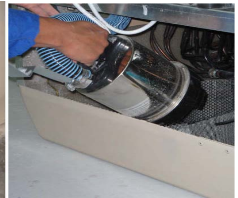
No need to remove pump's wiring Connection; only move pump to one side
