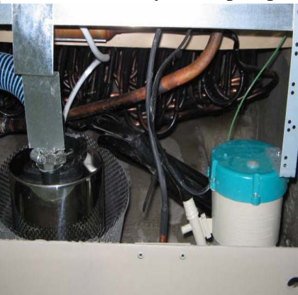
No need to remove pump's wiring Connection; only move pump to one side
