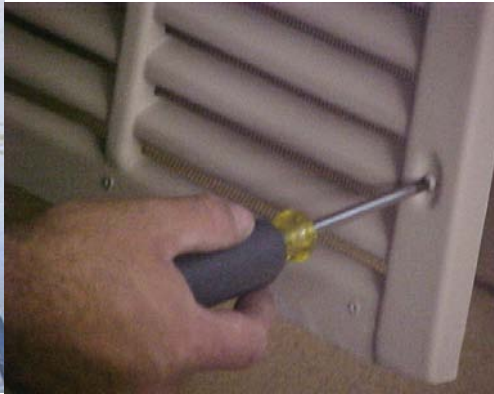
Remove the screened intake louver
