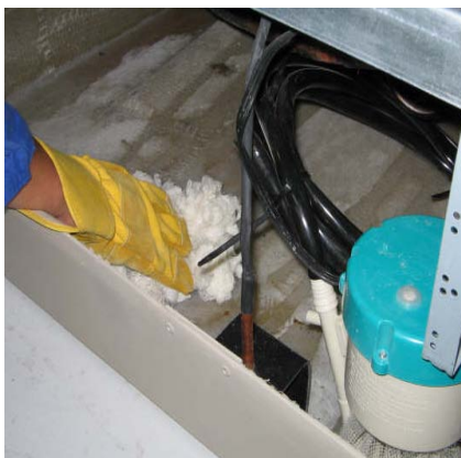
Remove pump & clean screen clean sump with a rag wearing gloves & eye guards.
