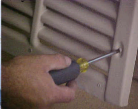
Disconnect All Electricity Before Servicing Remove the screened intake louver To avoid Electricity DANGER Of Serious Injury or Death
