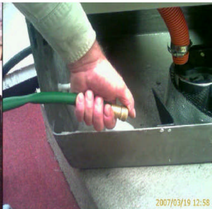
Rinse sump with Hose Reinstall Pump.
