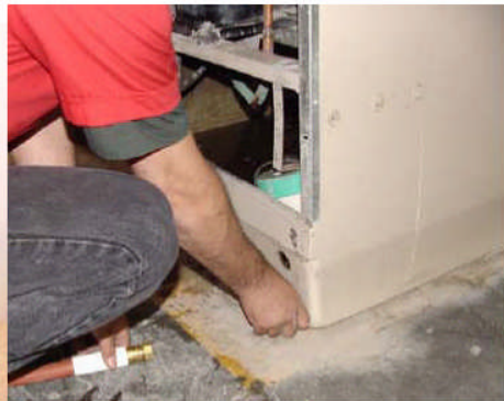
If desired, use a standard water hose to drain water to another location.
