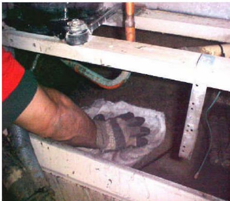
clean sump with a rag wearing gloves & eye guards.
